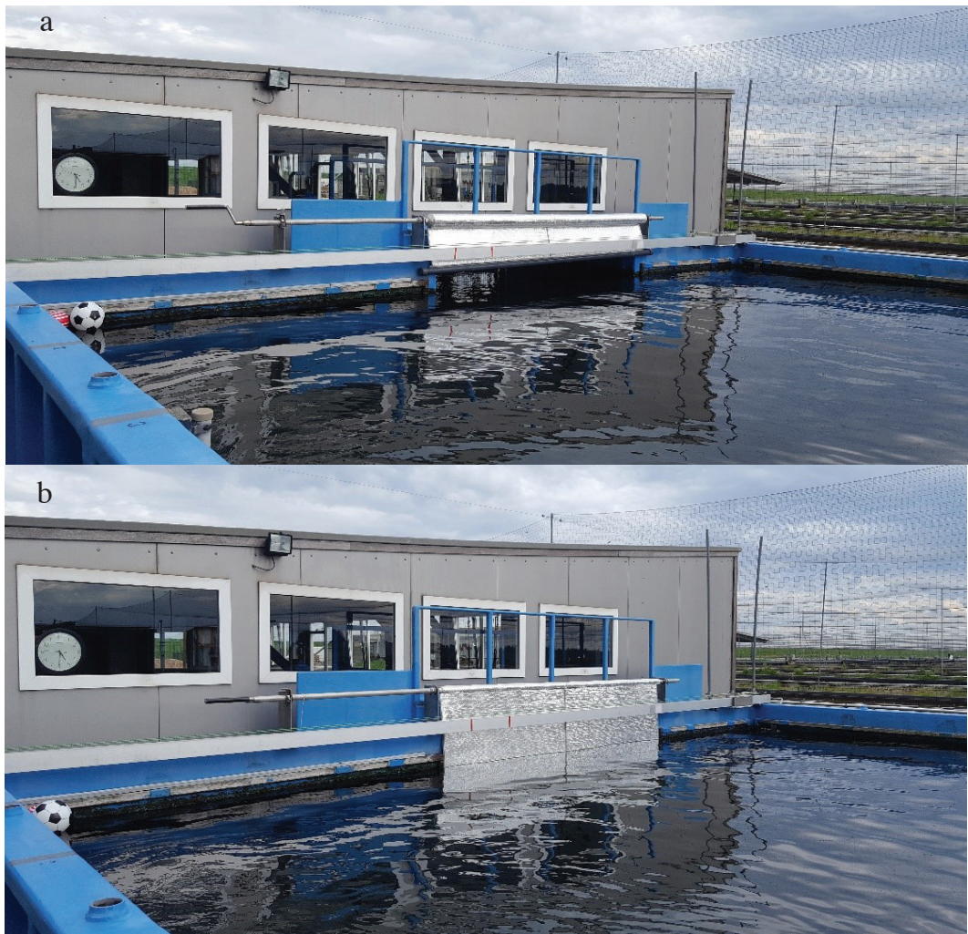
Figure 2. (a) The bubble screen rolled up above the water, and (b) the bubble screen deployed in front of the channel leading to the indoor pool
