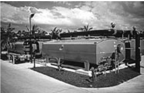
Figure 6.3. Horizontal steel filters
