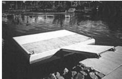
Figure 5.34. Floating platform with ballast system
