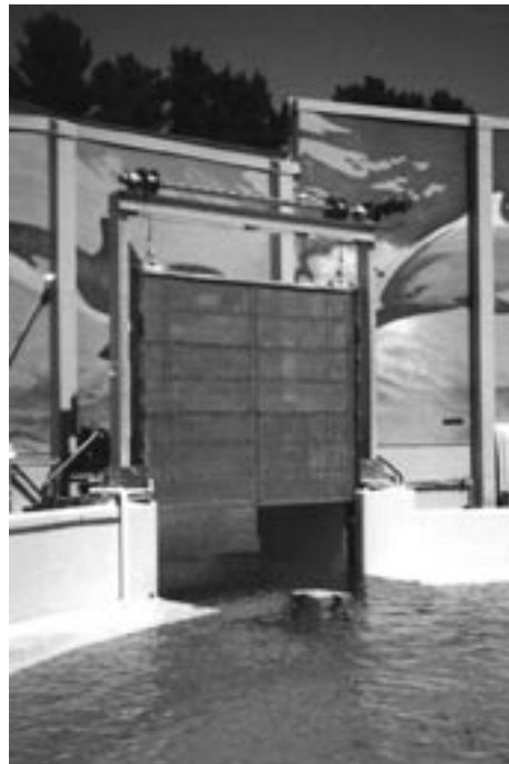
Figure 5.44. Vertical sliding waterproof gate
