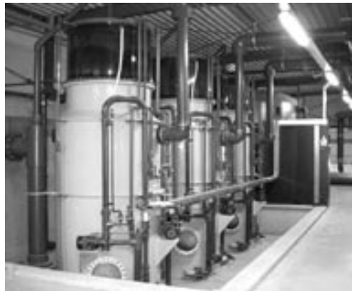
Figure 6.5. Protein skimmers with ozone injection (Photograph from I. Smit)
