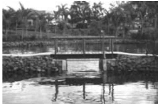
Figure 5.46. Rotating pneumatic gate with horizontal axis
