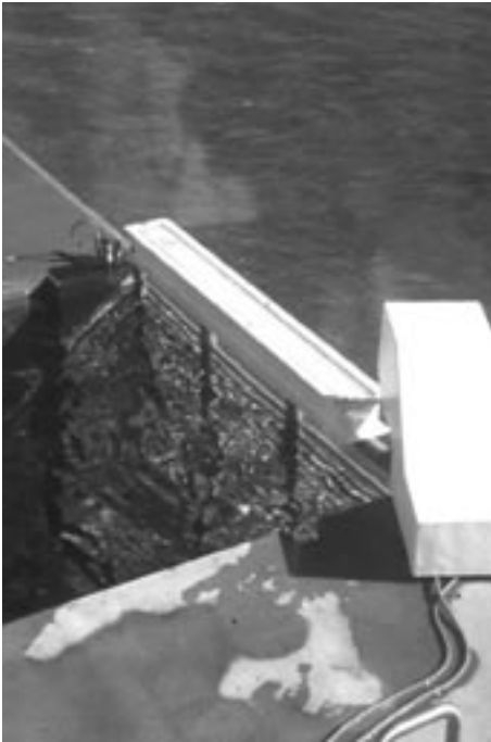
Figure 5.47. Rotating pneumatic gate with vertical axis
