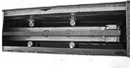
Figure 5.43. Horizontal sliding waterproof gate
