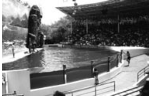
Figure 5.20. Artificial show facility
